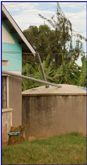
© Project WET Foundation Pictured: One of three new rain water harvesting systems at St. Kaggwa Primary School.
